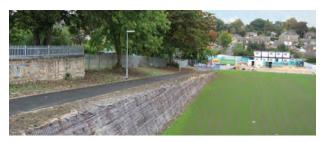
With construction successfully completed, the TensarTech GreenSlope can be prepared for the vegetation stage.
