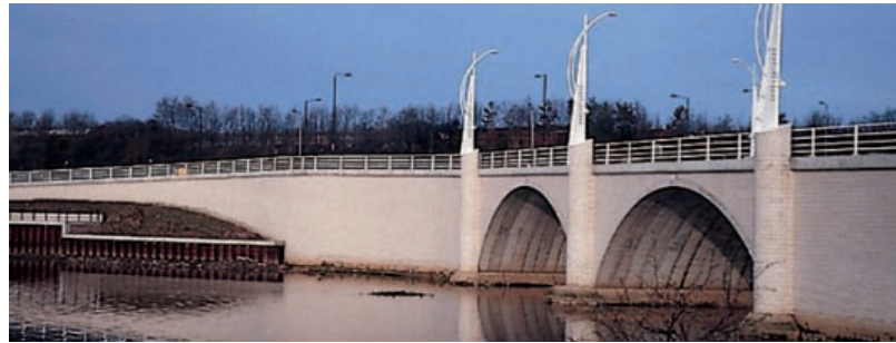
A modular block wall is used with spectacular effect on this twin arch bridge.
