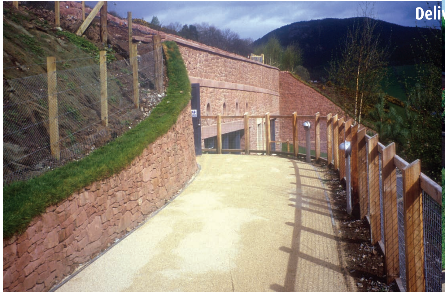
This sandstone finish was easily achieved by using a modular block wall system and stainless steel ties.
