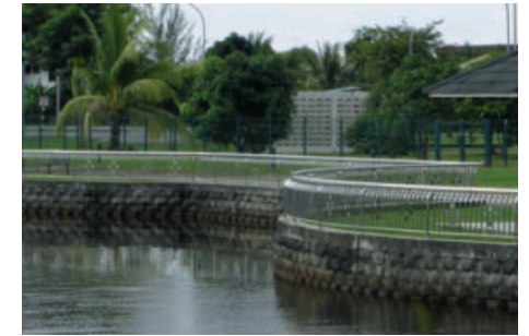
Tensar facing units provided the perfect solution in this marine location.
